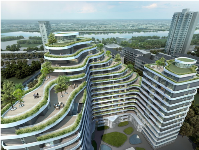
Shanghai Weifang Village Street project, Pudong District
