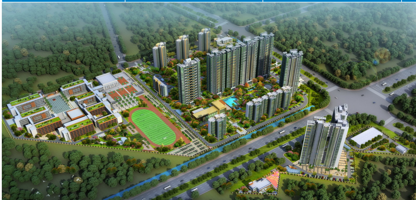
Phase 2 progress as of Feb 2016
