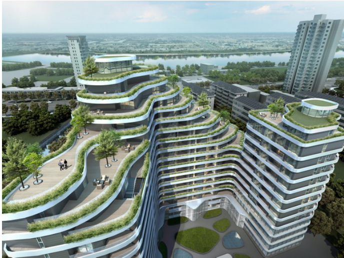
Shanghai Weifang Village Street project, Pudong District
