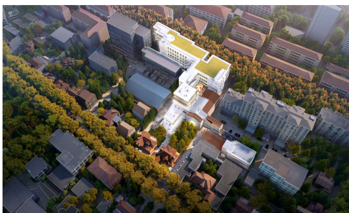
Shanghai Wuyi Road project
