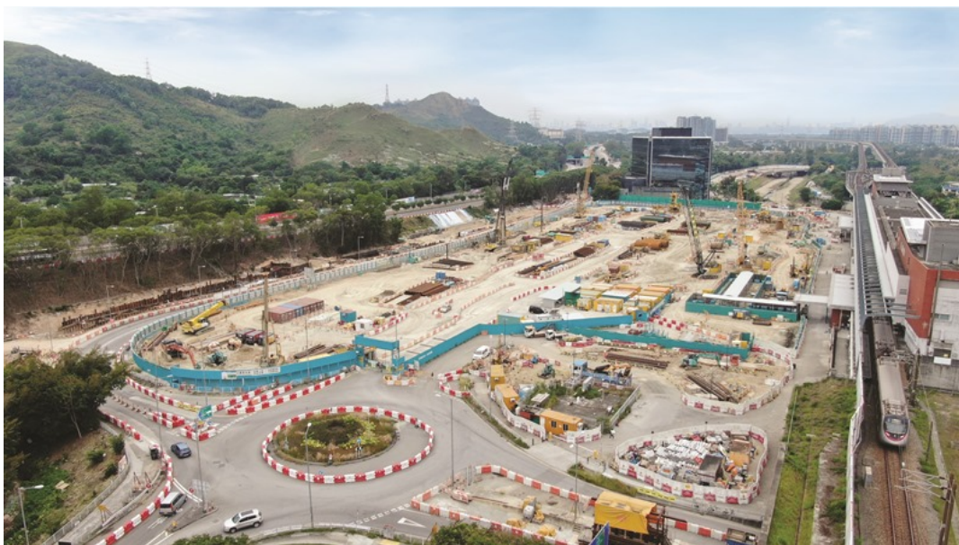
Kam Sheung Road Station, Yuen Long
